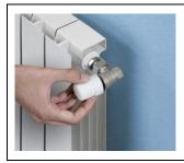
**1** - Remove the manual adjustment handwheel by loosening it anti-clockwise.
